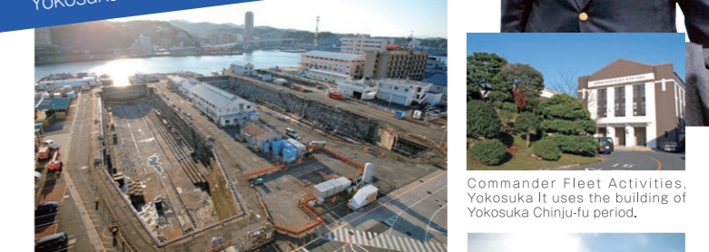
There remains precious heritage of modernization such as the dry dock built in Meiji through Showa era.
