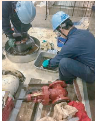
Cleaning each parts 各種部品の洗浄
